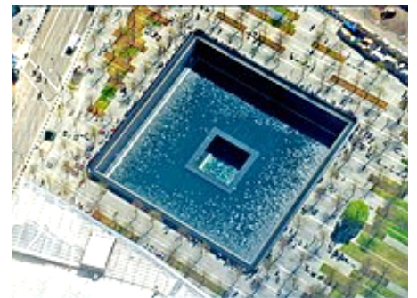
Aerial view of the South pool
